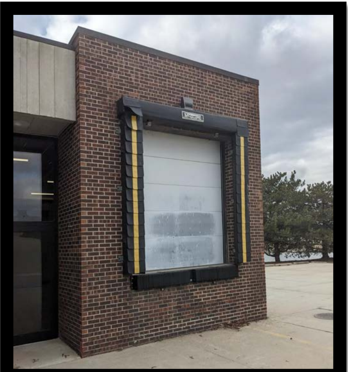
Dock and Stage Doors
